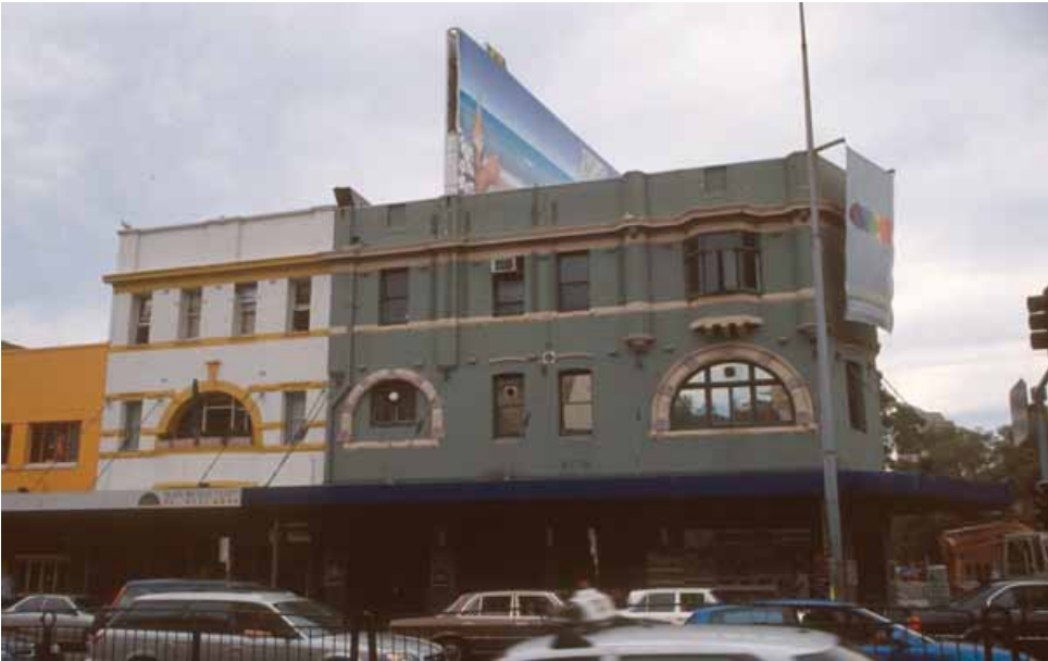
Photo showing the state of the external built fabric of 130-132 and 134 Oxford Street, Darlinghurst. The external fabric has undergone some changes like the removal of the higher corner parapet above the building's south facing chamfered corner. However, the overall external fabric has remained generally intact. The old McClrath's building has been replaced by a two-storey brick building painted in yellow as shown on the left of the photo. (Source: Mark Stevens Photograph Collection, City of Sydney Archives)
