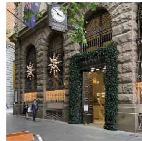
Fig. 6.2253 An adjacent former window now provides direct access to 2 Martin Place while the original corner stepped entry was kept intact. Internal refurbishment of ramp/lifts enable access to ground floor.
