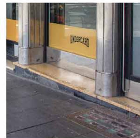
Fig. 6.2246 The shopfront on 82 Oxford Street, Darlinghurst rests on sloping terrain which required a step to keep the ground floor level. Future development may be faced with accessibility issues.
