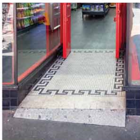
Fig. 6.2249 The shopfront on 103-105 Oxford Street, Darlinghurst exhibits a lower step-up from the sidewalk. The provision of a removable small ramp resolves the accessibility issue.
