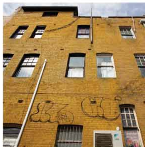
Fig. 6.2264 Exposed pipe work and electrical wiring on the Foley Street facing side of 108 Oxford Street, Darlinghurst
